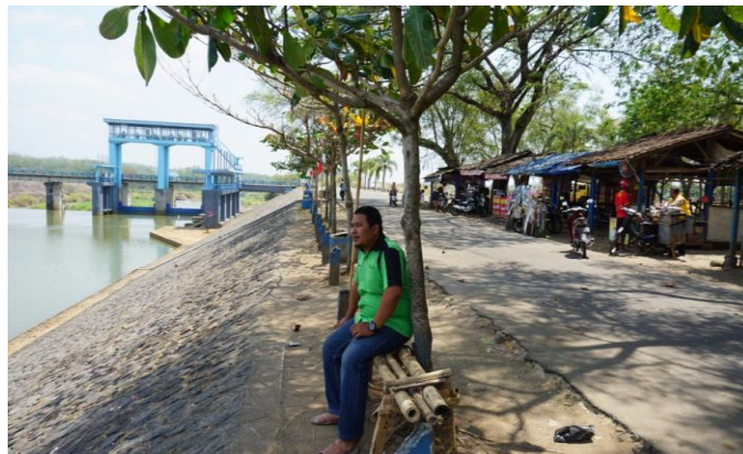
Figure1. DAM COLO location at Nguter Sukoharjo
