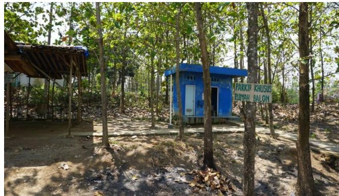
Figure1. The existing condition of toilet facilities
