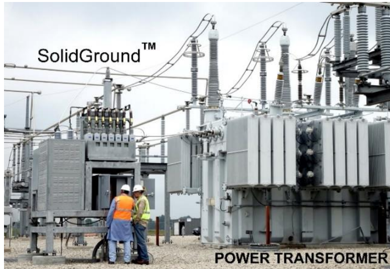
Figure6. Solid Ground™ by ABB (left) meant for blocking GIC in a neutral conductor of power transformer (right)
