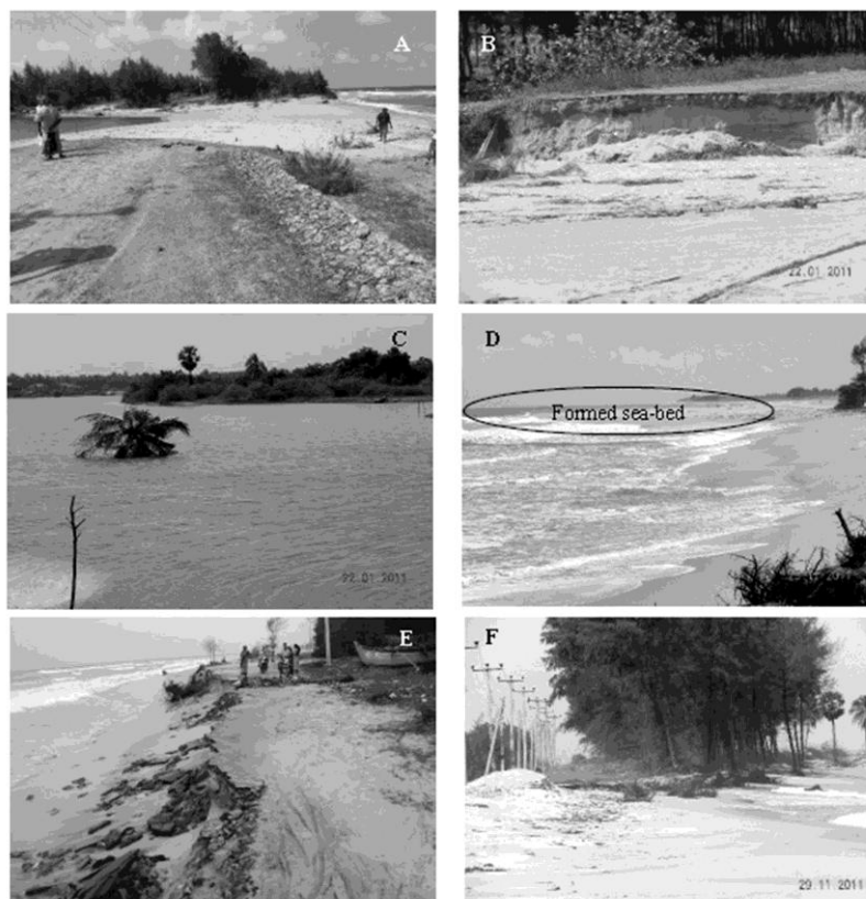
Figure3. Impacts of sea erosion due to man-made coastal opening at Navalady, Batticaloa. Extent of the opening increased by 70 times –estuary on left and the sea on right (A), about 2m depth of soil washed-off (B), private lands gone to estuary (C), opening led to formation of sea-bed (D), 600 m road washed off (E), planted Casuarina eroded (F). Photos: Mathiventhan, T (2011)
