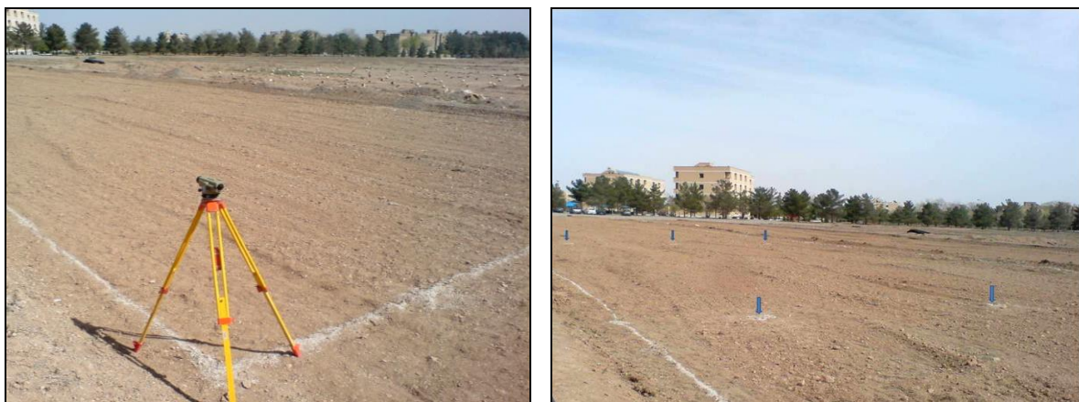
Fig 3. Field boundaries; Field surveying and gridding after initial leveling
