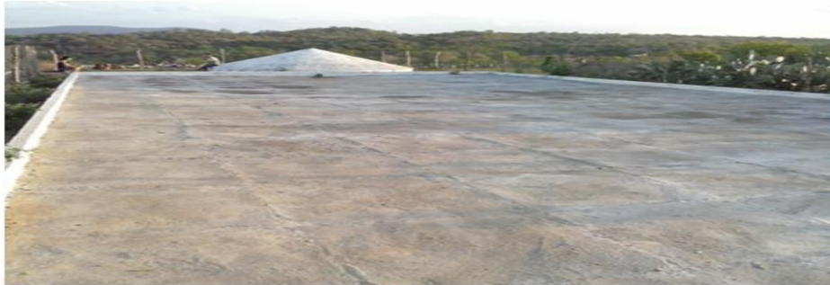
Figure2. First Boardwalk, Built in Cement Soil, to Capture Rainwater in Barra De Santana, Paraíba, Brazil
