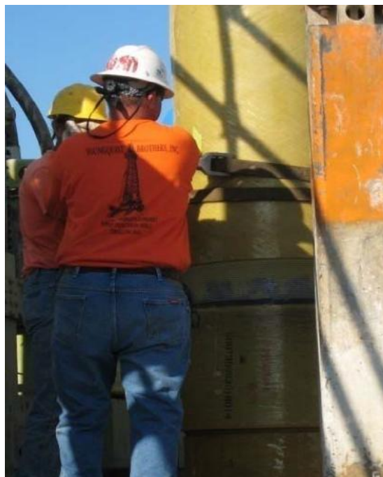
Figure9. Use of Strap Wrenches with Fiberglass Casing, courtesy of Future Pipe Industries
