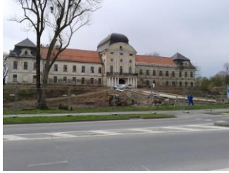
Works on reconstruction of the Pejačević Castle
