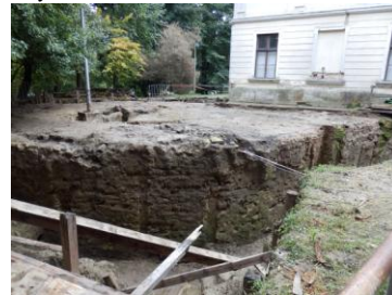
The foundation of north- east tower
