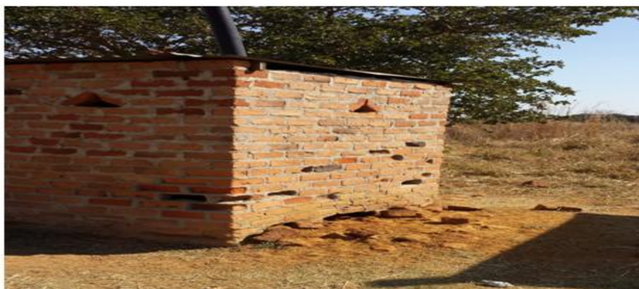
Picture1. A School pit latrine vandalised by pigs following the salty urine
