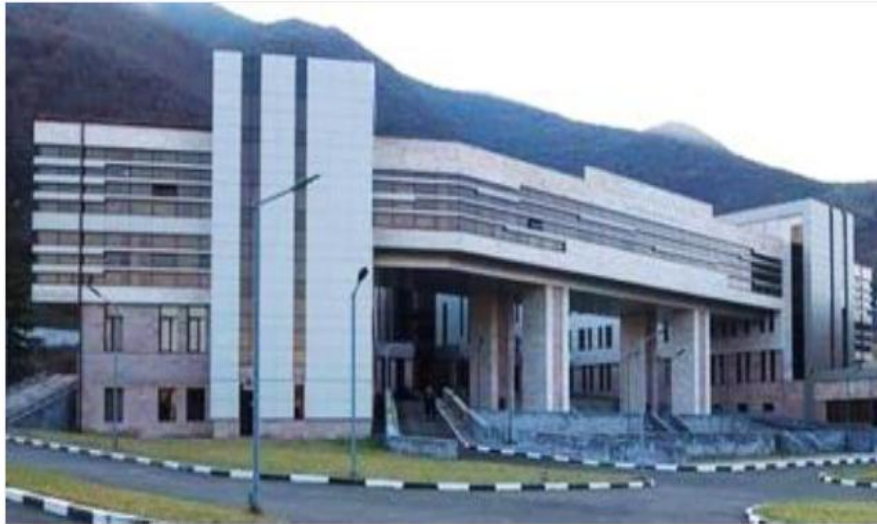
Figure13. View of the 4-story base isolated hospital building “Vanadzor” after completion of construction
