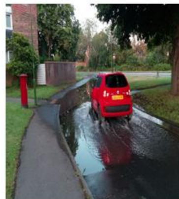
Fig4. No Drainage at all
