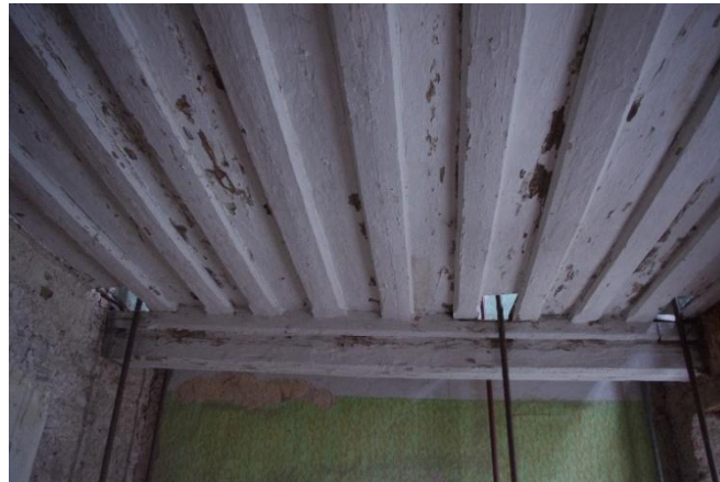
Figure2. Timber floor bottom view
