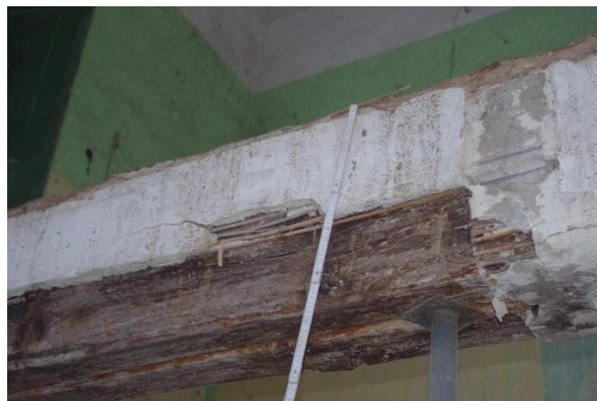
Figure3. Timber beam with a reed plaster
