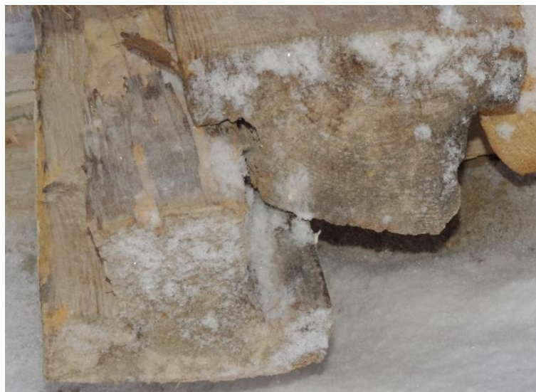
Figure 6. Timber joist cross section (already demolished floor)
