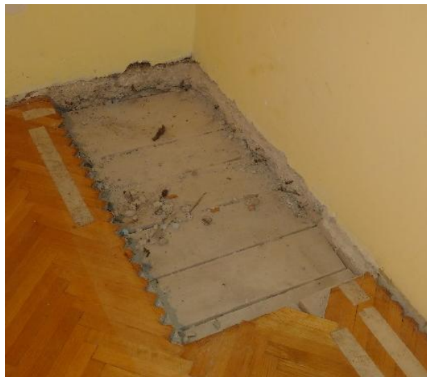
Figure 1. Time consuming examination of a timber floor
