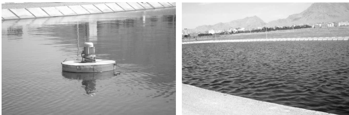
Fig1. Aeration and stabilization lagoons (left to right respectively)
