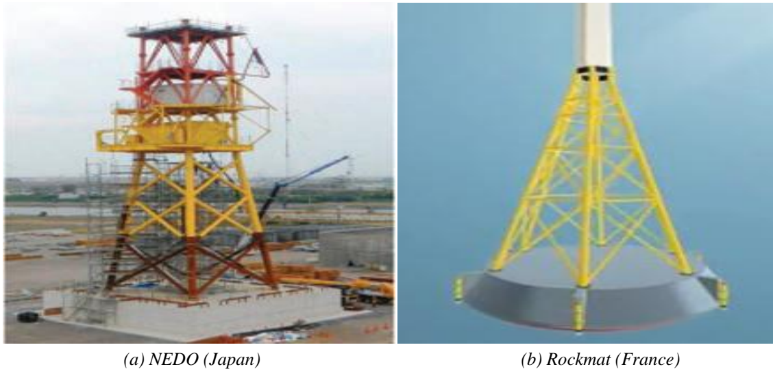
Fig1. Hybrid types substructure system
