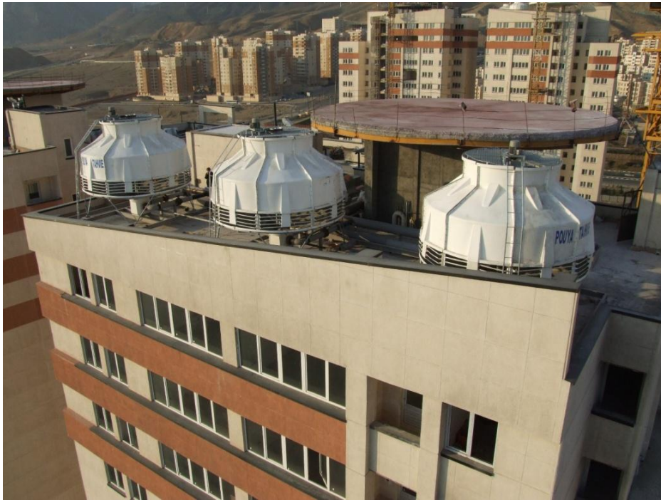
Figure1. A sample of the wet cooling towers on the highest location of a building
