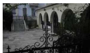
Fig11. The same Greek Orthodox Church as above, with the staircase going down 1.5 m. According to Eg. (1,1S).
