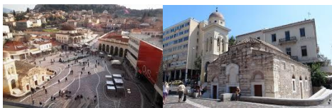
Fig14,15. Two photographs of buildings lower than street level, old Orthodox Church near Acropolis, Athens, Greece, Eg. (1,1S).
